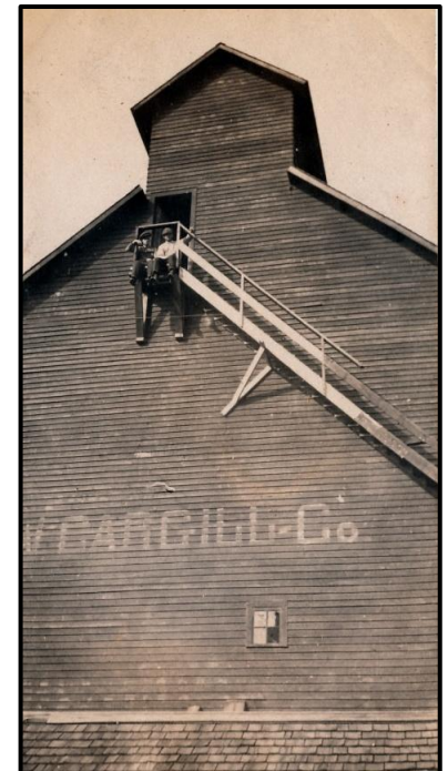
Cargill Grain Elevator
