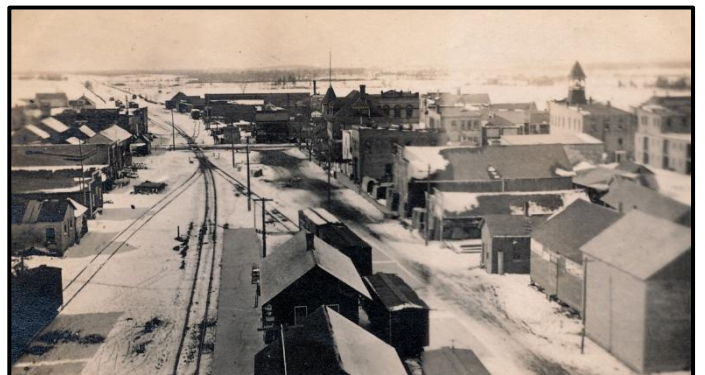
Looking west with the depot in the foreground. From the top of the Cargill Grain Elevator - 1914
